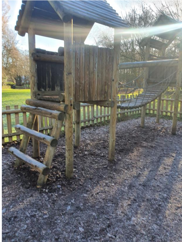
Repair agreed issues on existing towers
