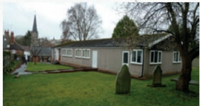
Baptist Hall, behind Baptist Church, High St.
