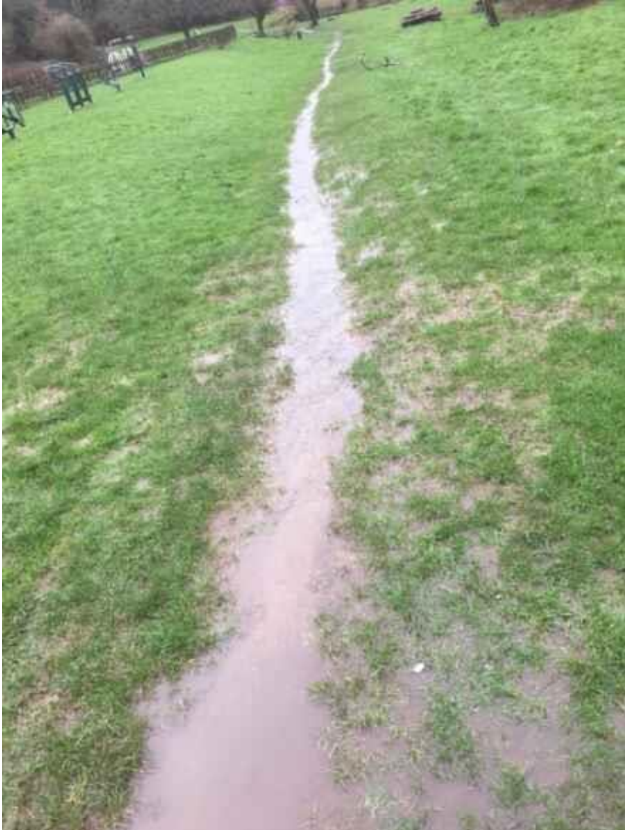
Water flowing down worn foot path towards lowest point
